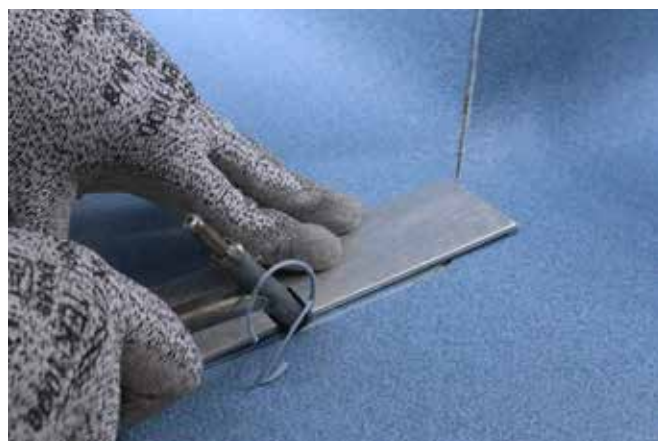
2. Groove the join on the flat section of the floor.
